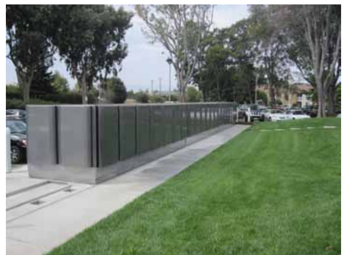
Business sized Solid Oxide Fuel Cell (BloomBox EnergyServer™) creating efficient green electricity using natural gas in California, USA
