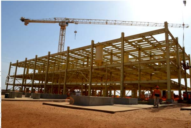
Dry mill construction at the MSP progresses
