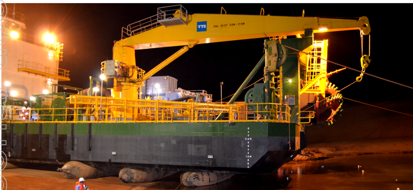
Dredge being winched into position mid-launch
