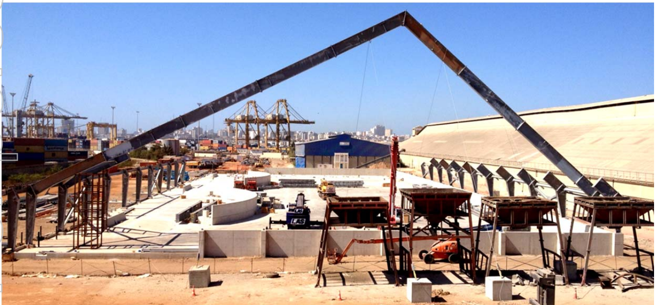
Concentrate warehousing under construction at the port
