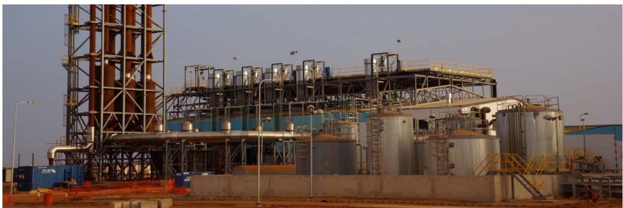
Power station construction complete with first engine started late March
