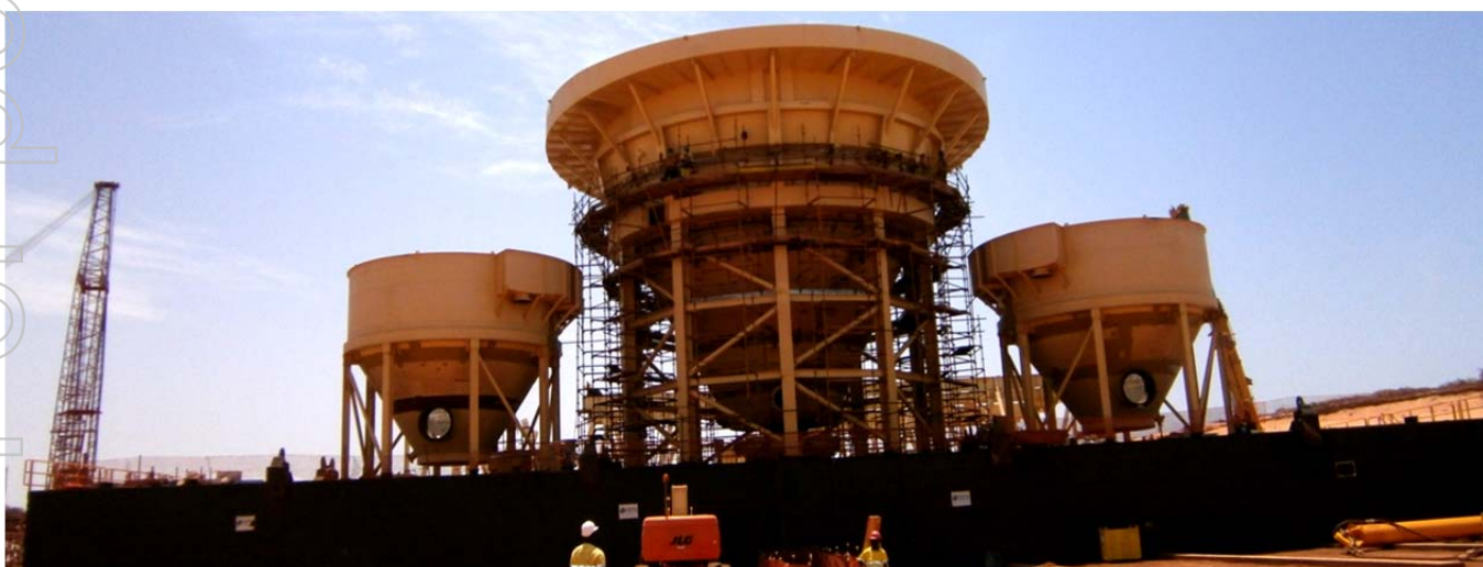
Surge bin is lifted into place on the WCP pontoons
