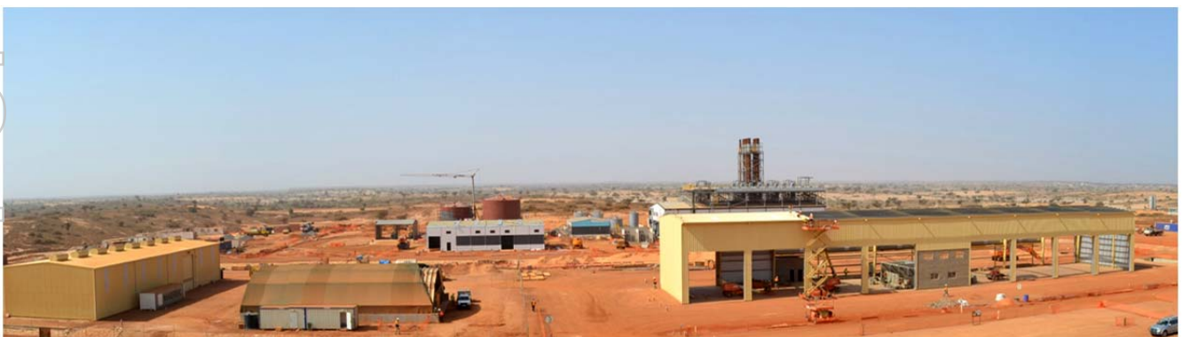
Construction at the MSP - stores (left) and workshop (right)
