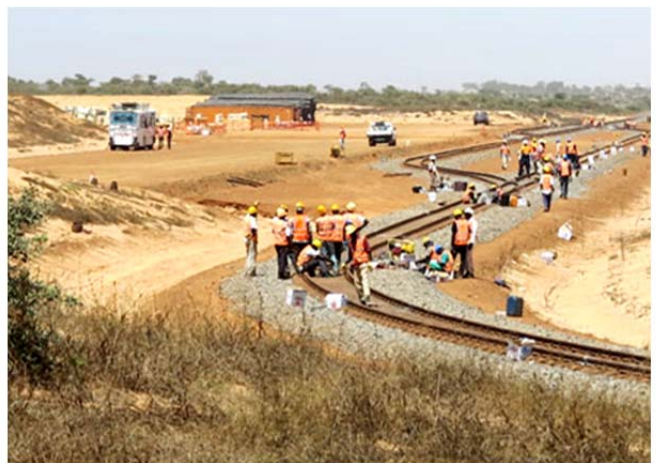
New track from the MSP to Mécckhe nears completion
