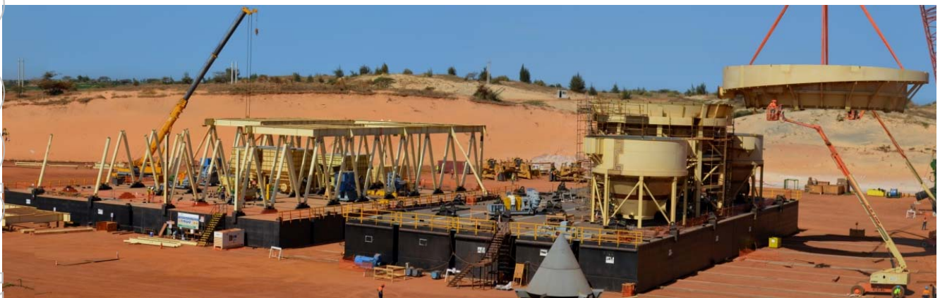
Construction of spiral module & surge bin assembly progresses at the WCP
