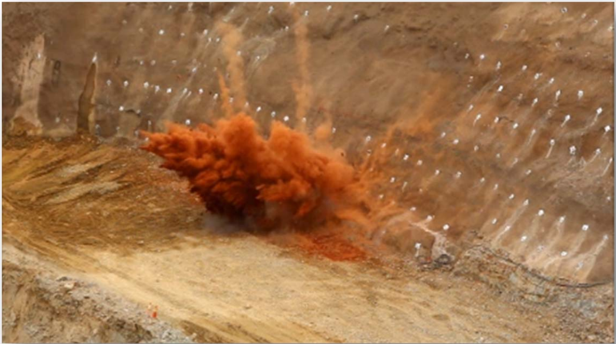
Figure 1. First portal trim blast to establish the underground access.
