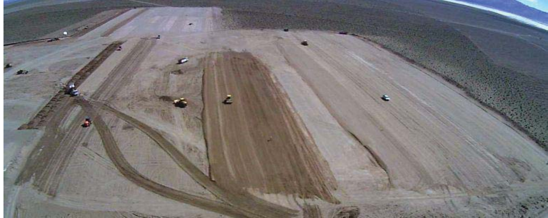
Aerial view of camp pad construction
