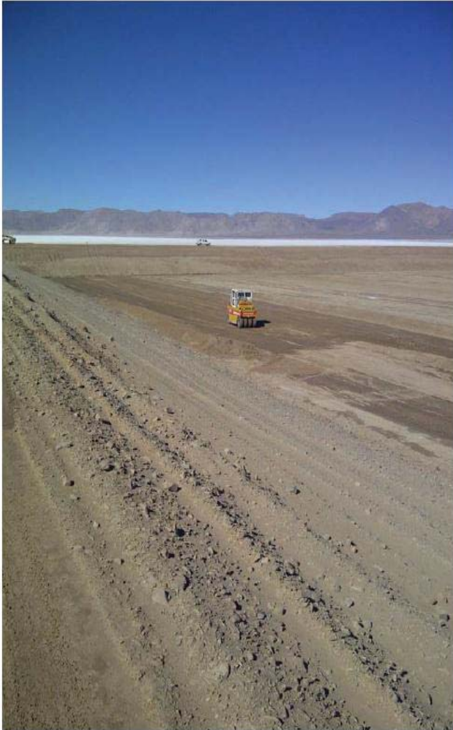
Evaporation Pond under construction
