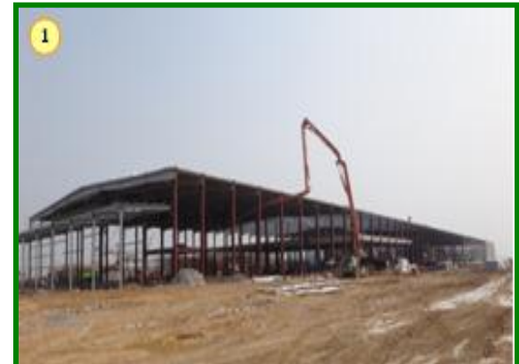
Most recent photographs of construction
