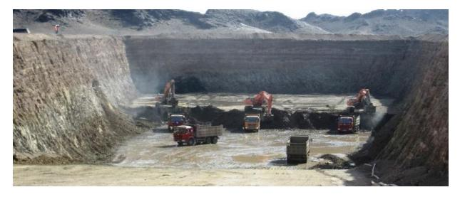
This photograph shows excavators benching down to top of coal. Overburden is trucked out and placed in an out-of-mine waste dump
