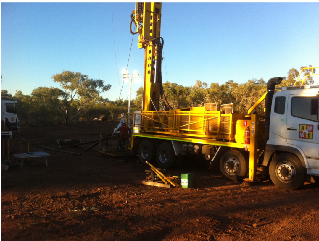
Figure 1: Diamond drill hole LBD4 in progress
