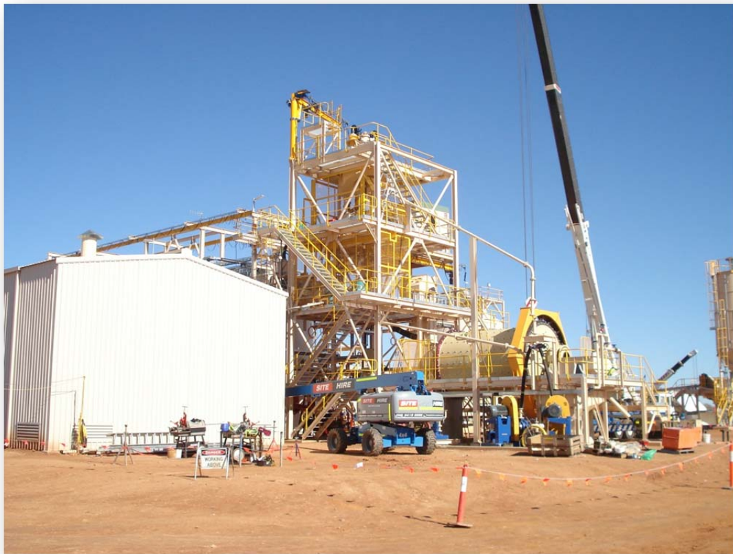
Figure 3. Ball mill and gravity circuit installation progress.
