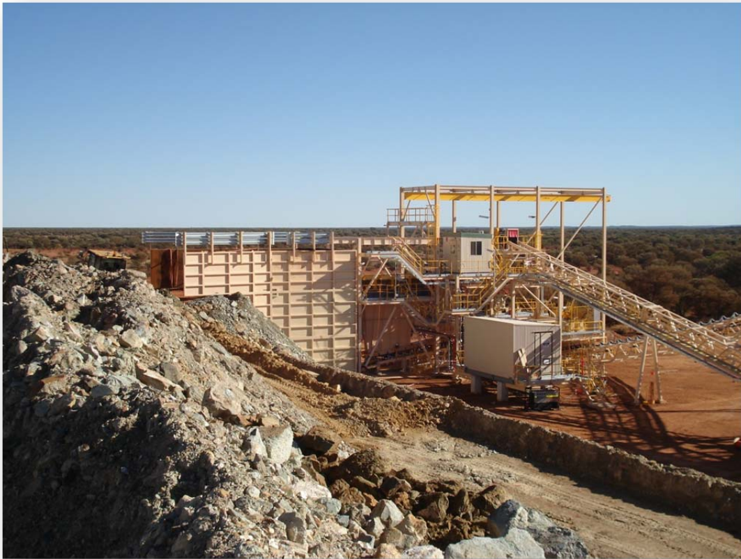
Figure 7. ROM grizzly feed into primary crusher nearing completion.
