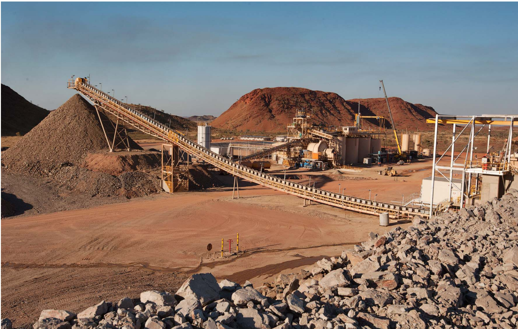
Process Plant: View from ROM Pad
