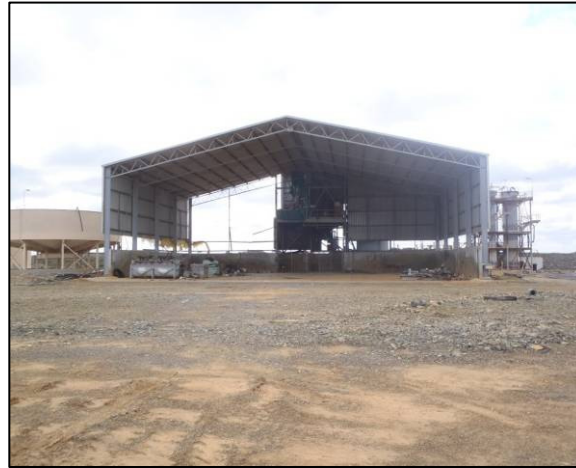
Concentrate thickener & concentrate storage shed at Rav 8
