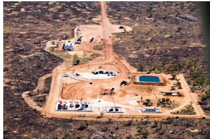
Aerial view of current Ungani Oilfield facilities
