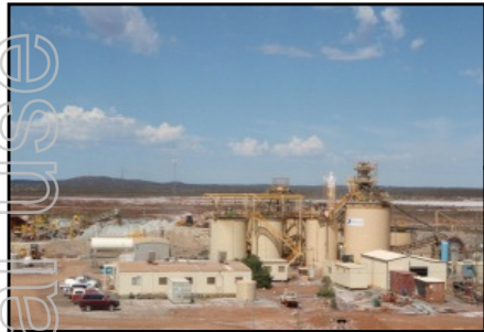
Lakewood Mill (800-900kt pa)
