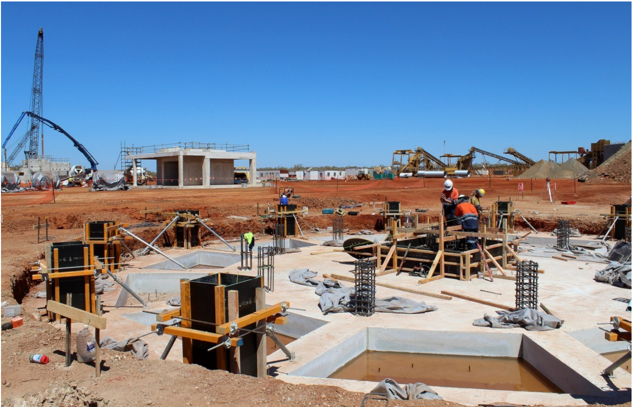
Figure 3: Foundations for the tailings thickener.
