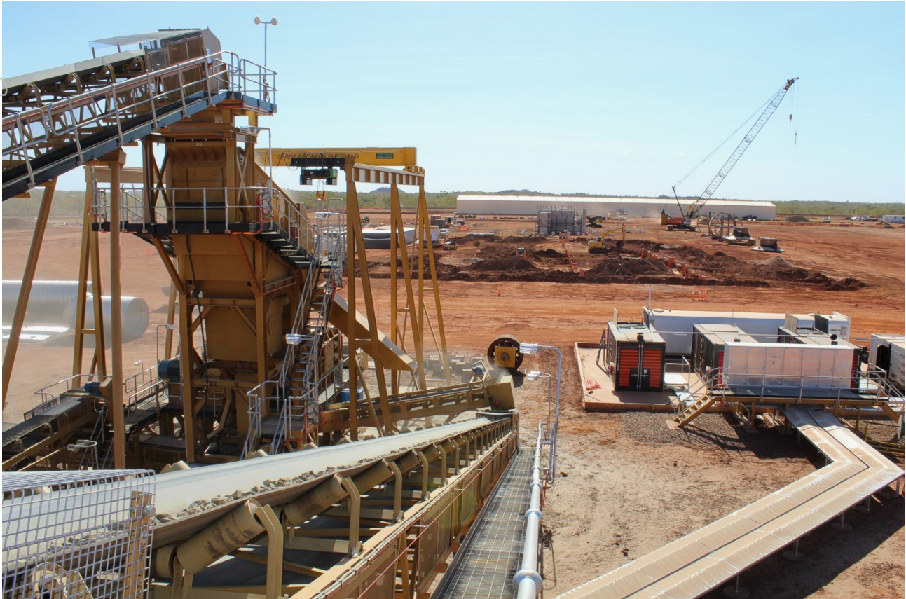
Figure 8: The crushing circuit undergoing commissioning (foreground), major earthworks commence at the site of the gravity circuit (middle distance), concrete foundations for the ball mill (background) and Process Plant Stores shed (far background). The site of the HPGR is obscured by the crushing circuit (middle distance to the left of the image).
