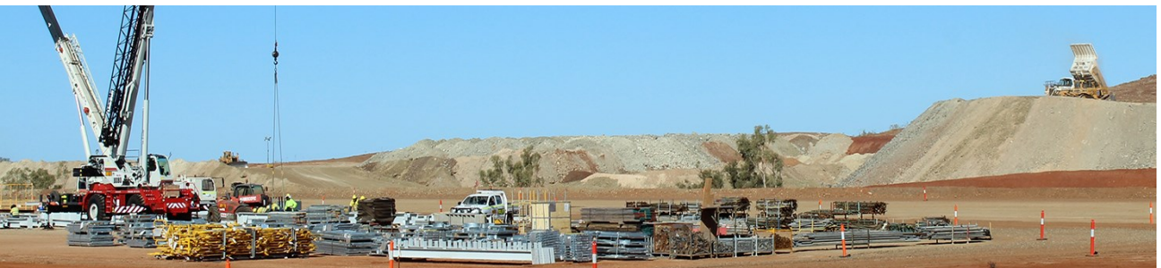
Figure 14: Various plant and equipment components arrive at site.
