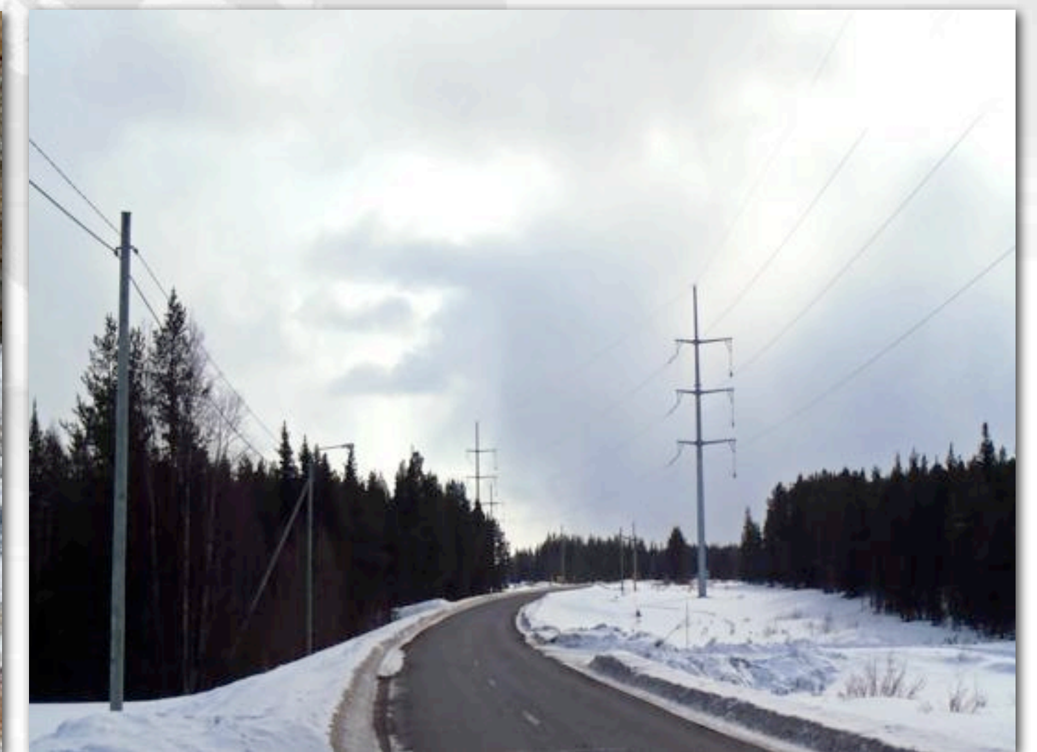
Road and grid power running through project
