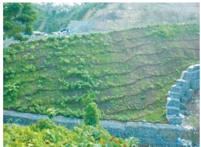
Photo 9: Revegetation on Slopes
