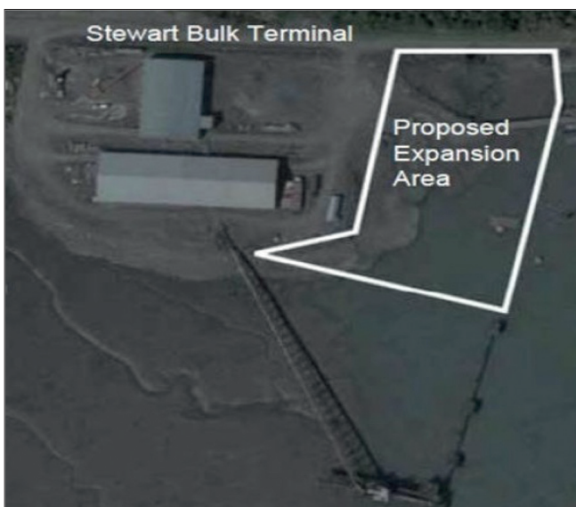
Stewart Bulk Terminal proposed expansion site
