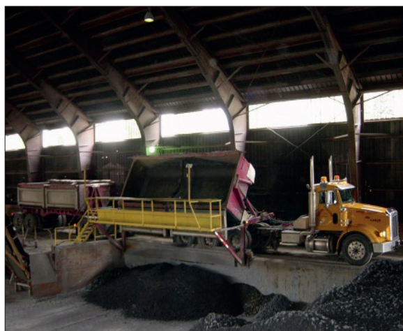
Stewart Bulk Terminal existing storage facility
