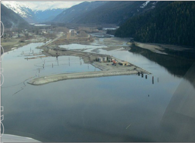
Stewart World Port dock under construction
