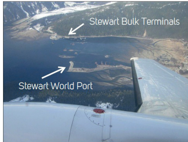
Stewart World Port dock aerial view
