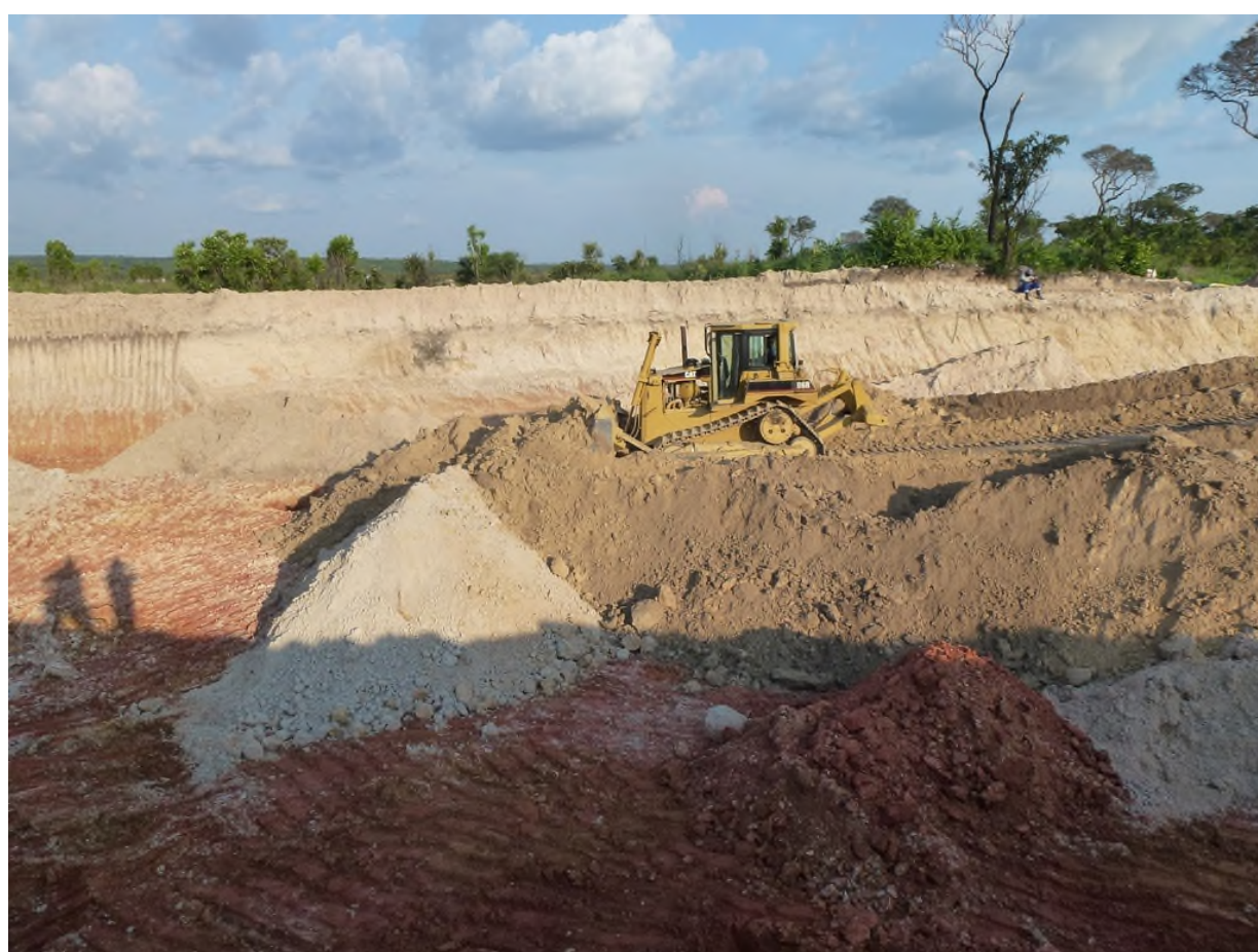
Pit excavation work at the Lulo Diamond Concession
