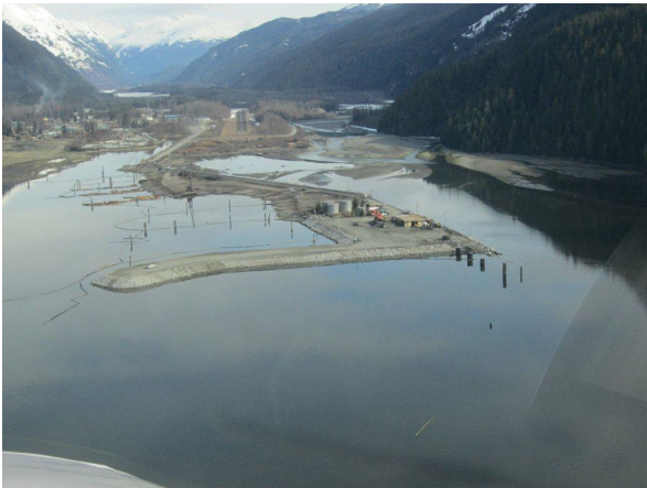
Stewart World Port dock under construction
