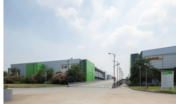
Goodman Waigaoqiao, Distribution Centre, Shanghai, China
