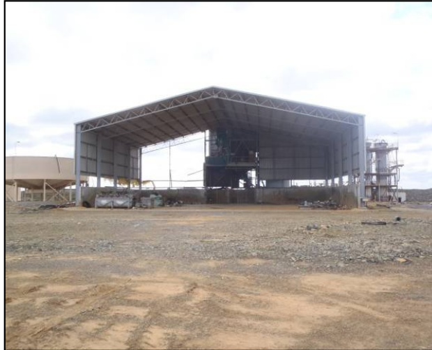
Concentrate thickener & concentrate storage shed at Rav 8
