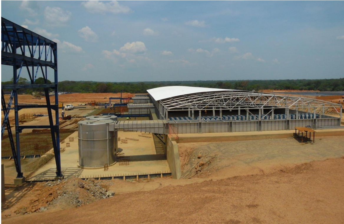
Solvent Extraction module ready for dry commissioning
