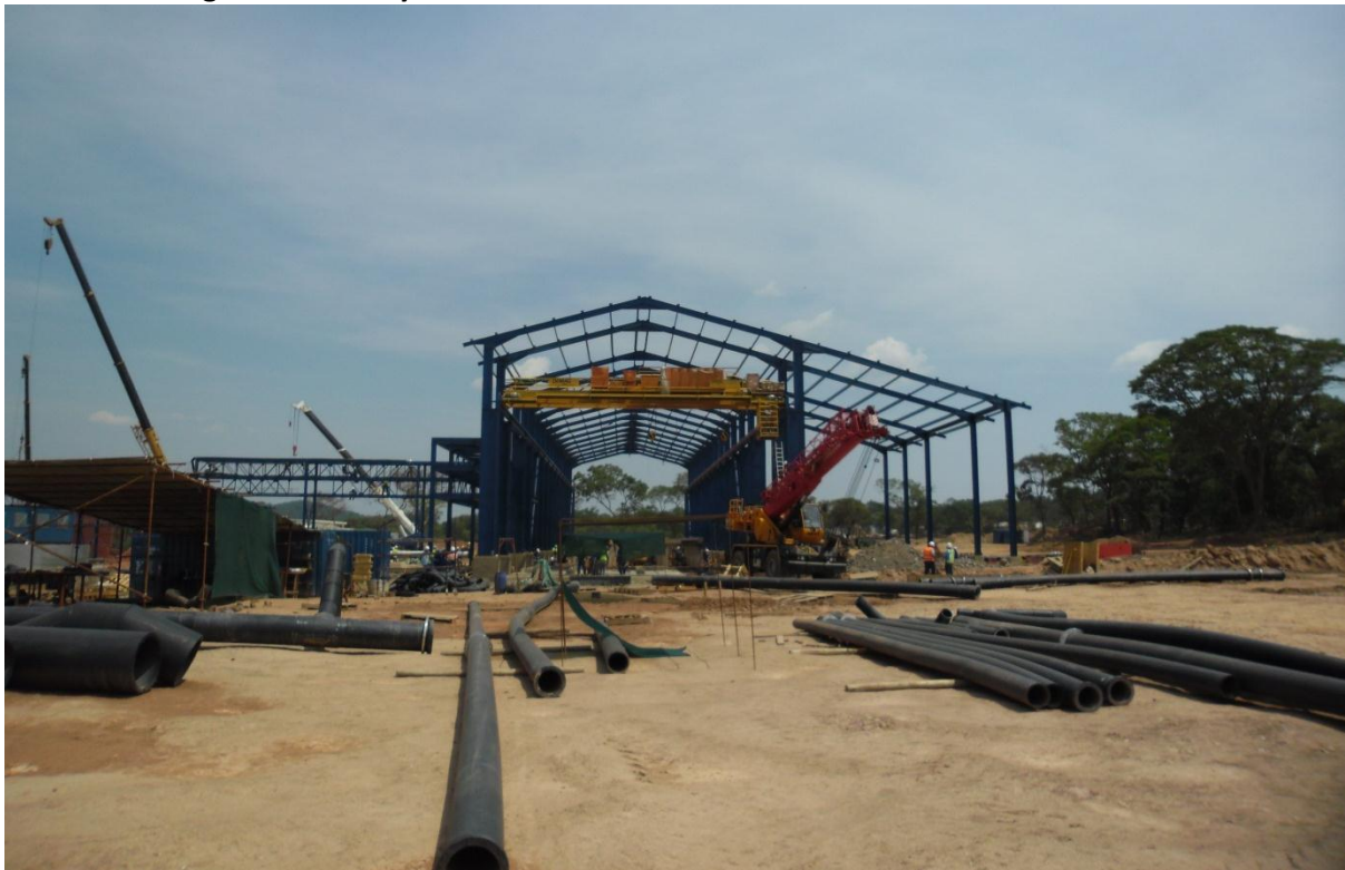
Electro-winning module ready for roof installation
