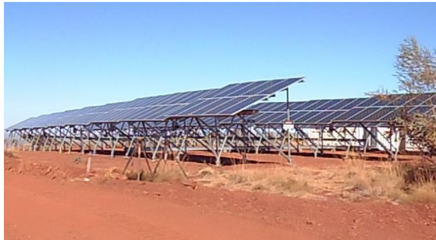
BHP Remote Area Power Station – Hybrid diesel/ solar/ battery
