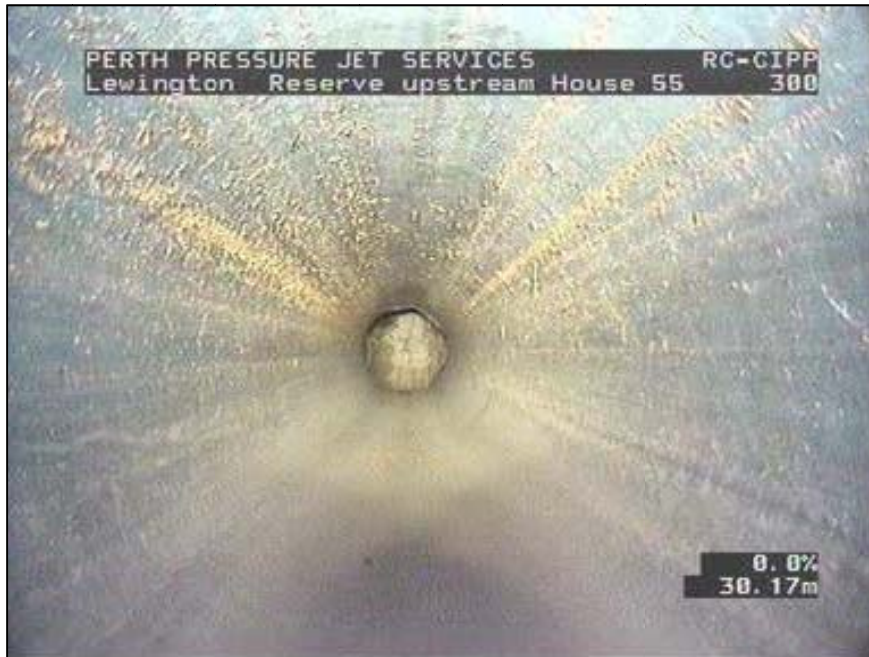
Image 2: Storm water pipeline in City of Rockingham, November 2013
