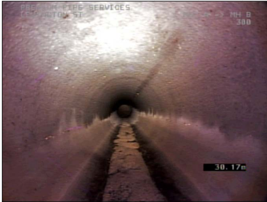
Image 1: Storm water pipeline in City of Rockingham, December 2008
