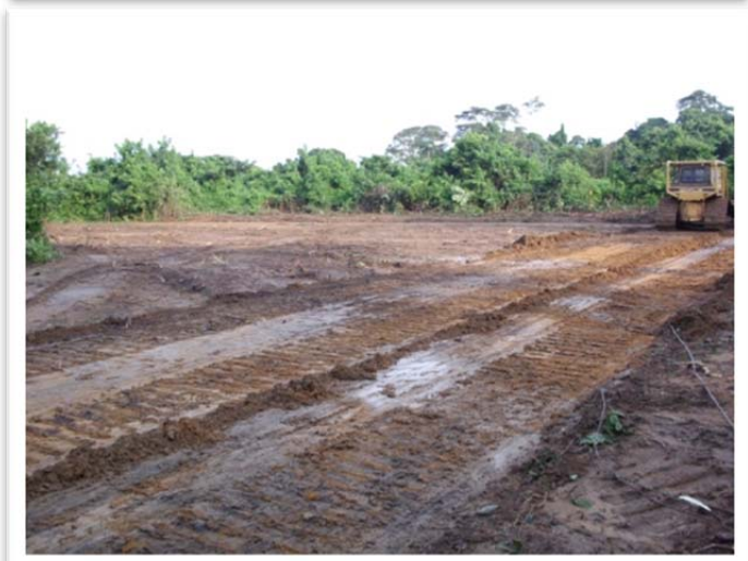
Photos from site clearing preliminary works undertaken at the location of the Lolabe Mineral Terminal in December 2013
