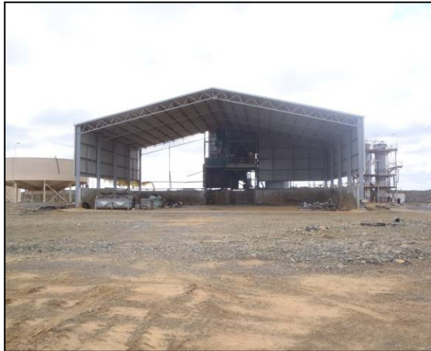
Concentrate thickener & concentrate storage shed at Rav 8
