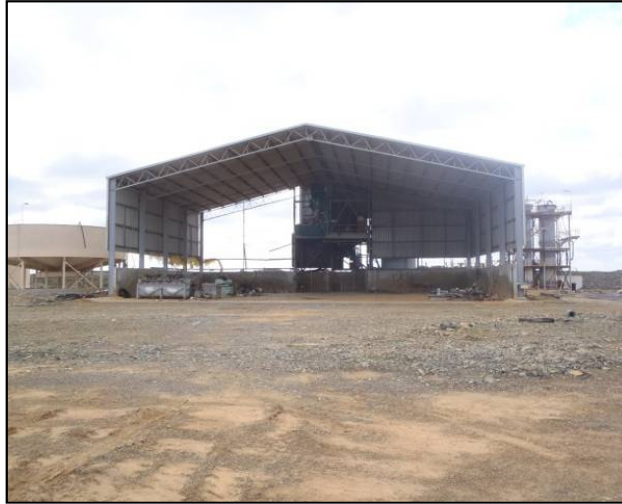
Concentrate thickener & concentrate storage shed at Rav 8
