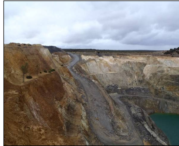
Rav 8 open pit - Potential In-Pit Tailings Storage Facility
