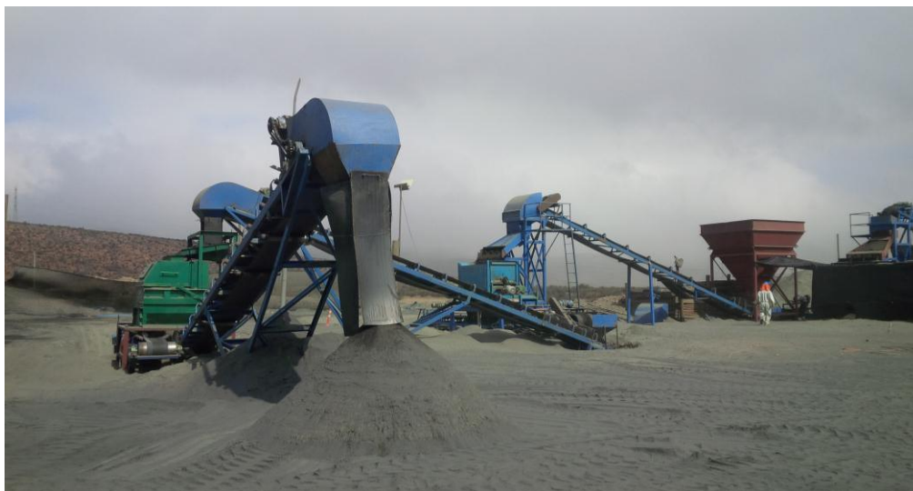
Figure 1: Final Magnetite Concentrate Produced During the Commercial Trial
