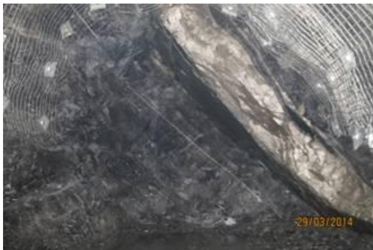
1020 Ore Drive: Split fired drive face after bogging of the waste rock
