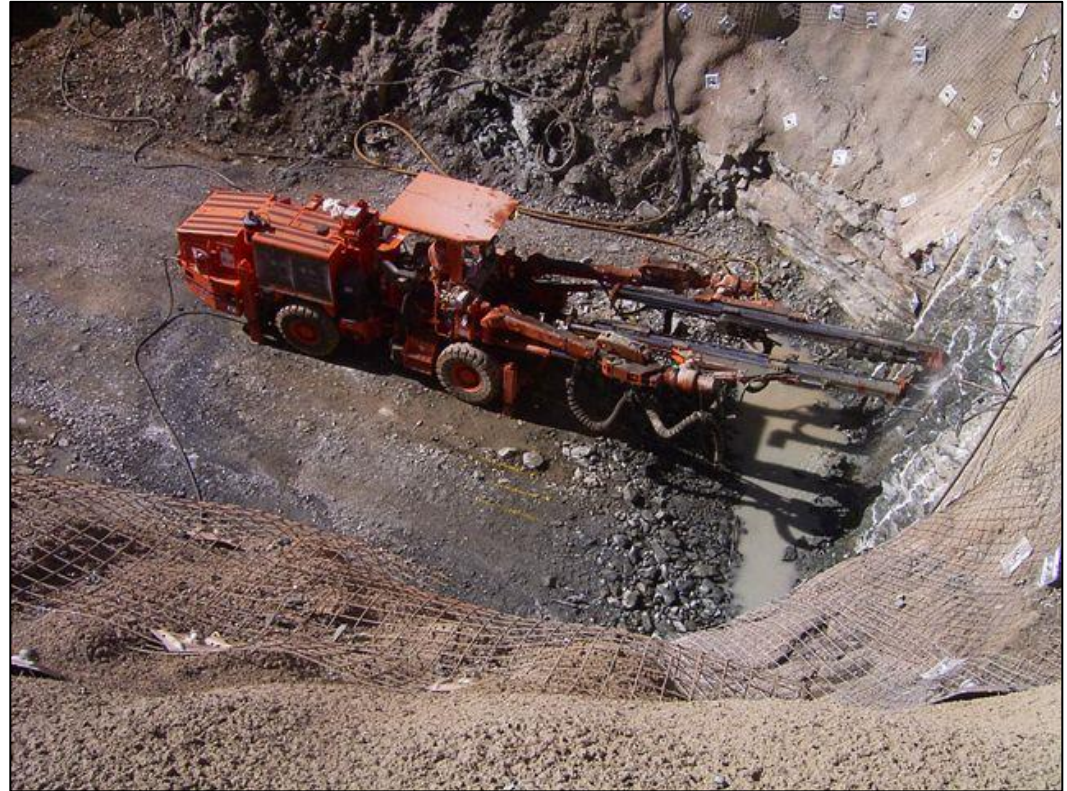
Jumbo drilling boxcut at Winner
