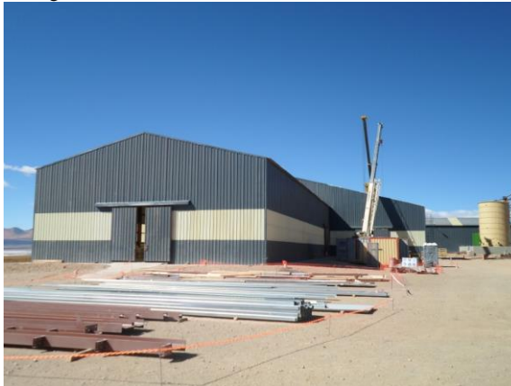
Dense soda ash warehouse
