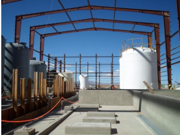
Lithium carbonate plant
