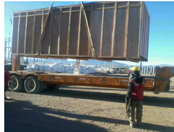
Equipment delivery to site
