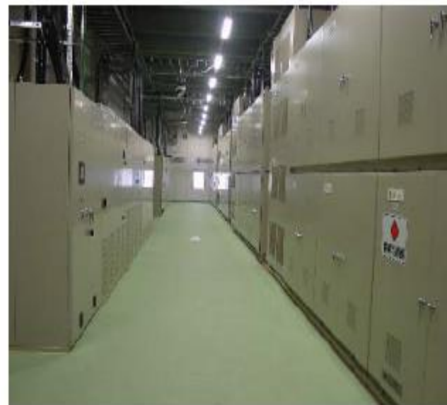
VRB cell stacks at Tomamae Wind Farm, Japan (Source: J-Power)
