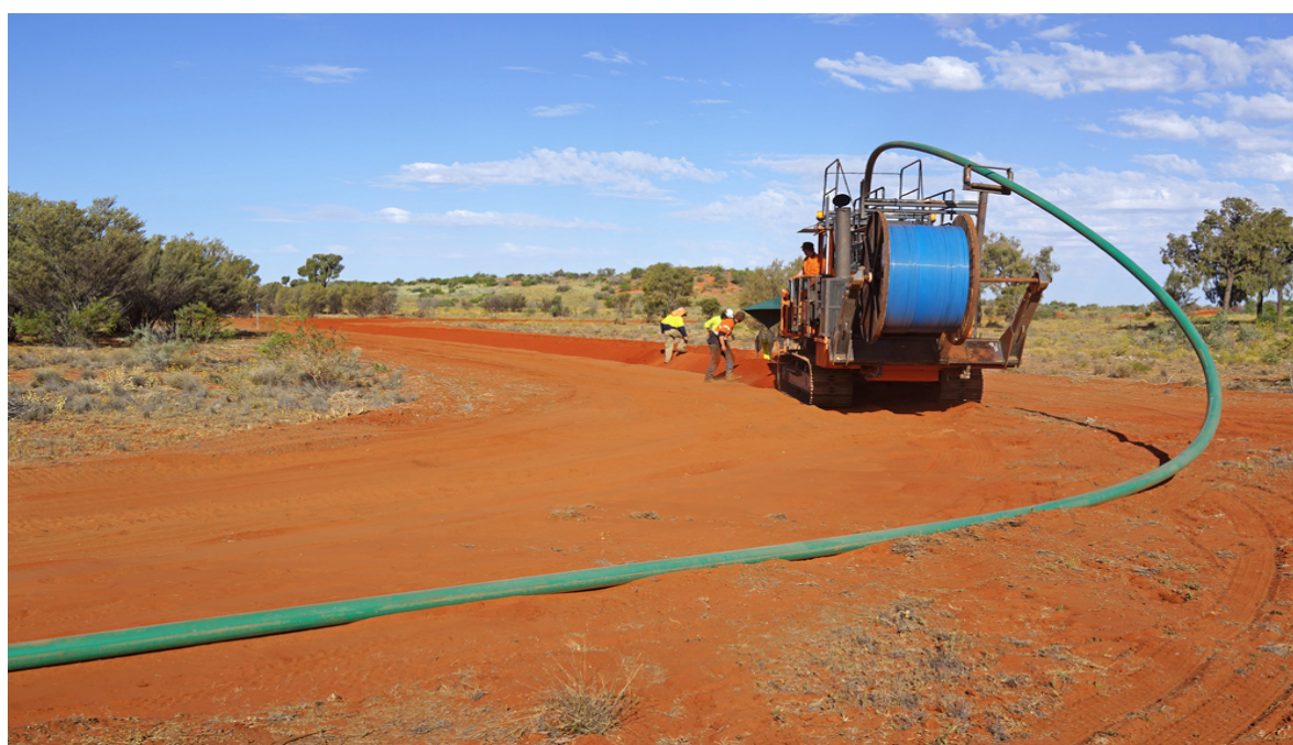
Laying the Dingo Gas Pipeline near Alice Springs, Northern Territory
