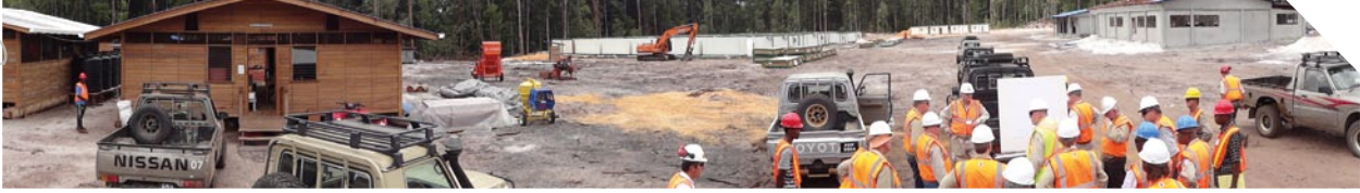
Camp Site Construction - Karouni, Guyana
