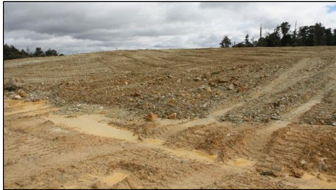
Nov 2013, Final re-contoured profile of the Settlement Dam waste stockpile
