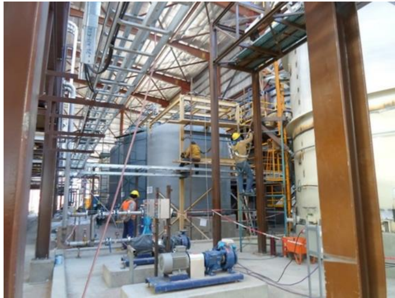
Construction of the lithium carbonate plant
