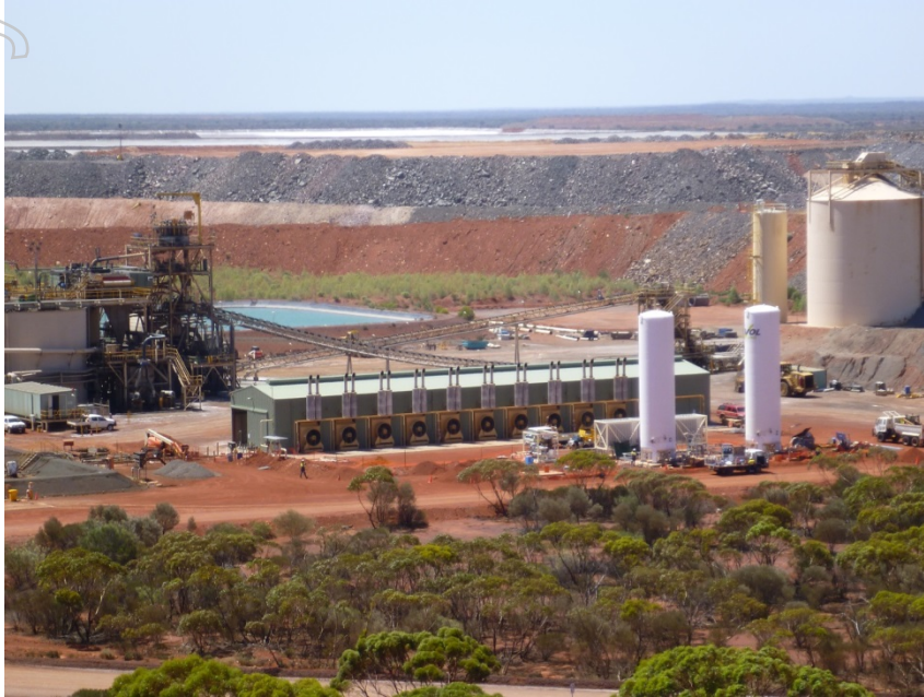
Figure 12 – LNG storage and vaporisation facility in the foreground of the power station
