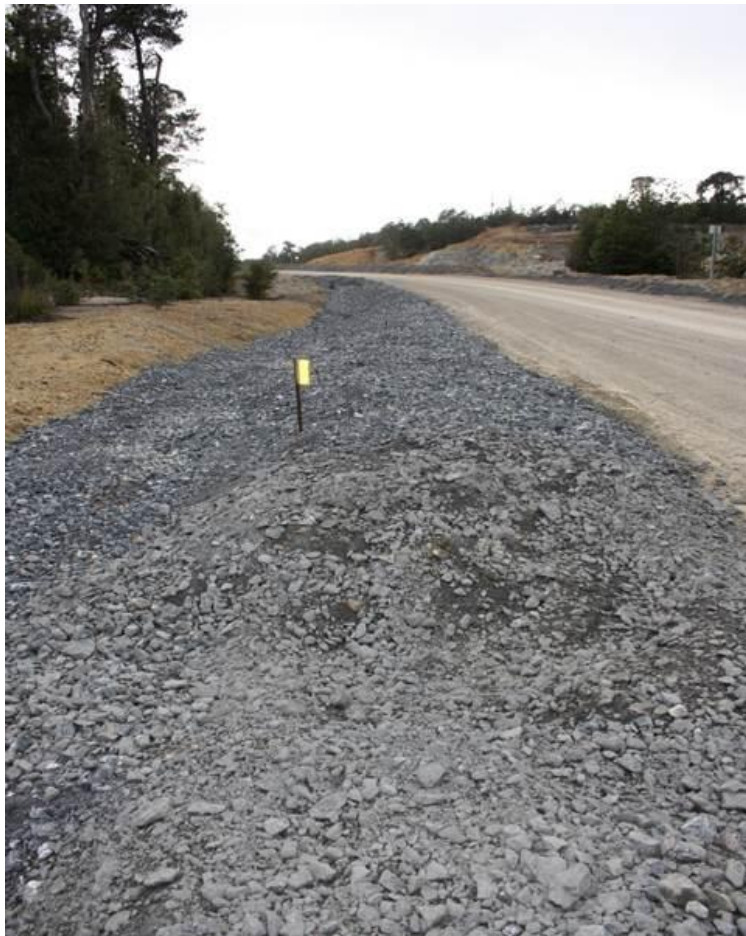
Drains and windrows lined with Limestone to improve pH
