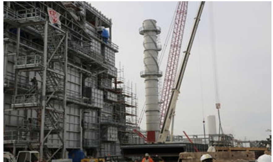
Secondary reformer crane pad being prepared
