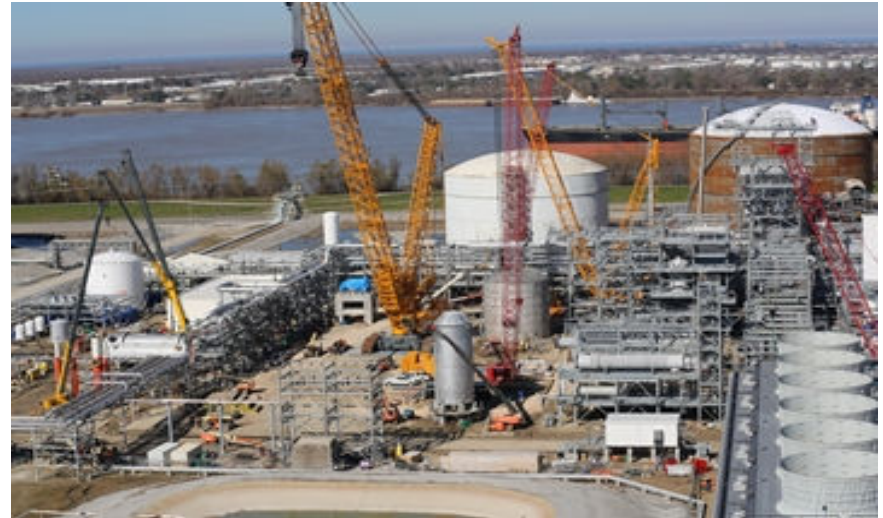
Overall construction view looking North
