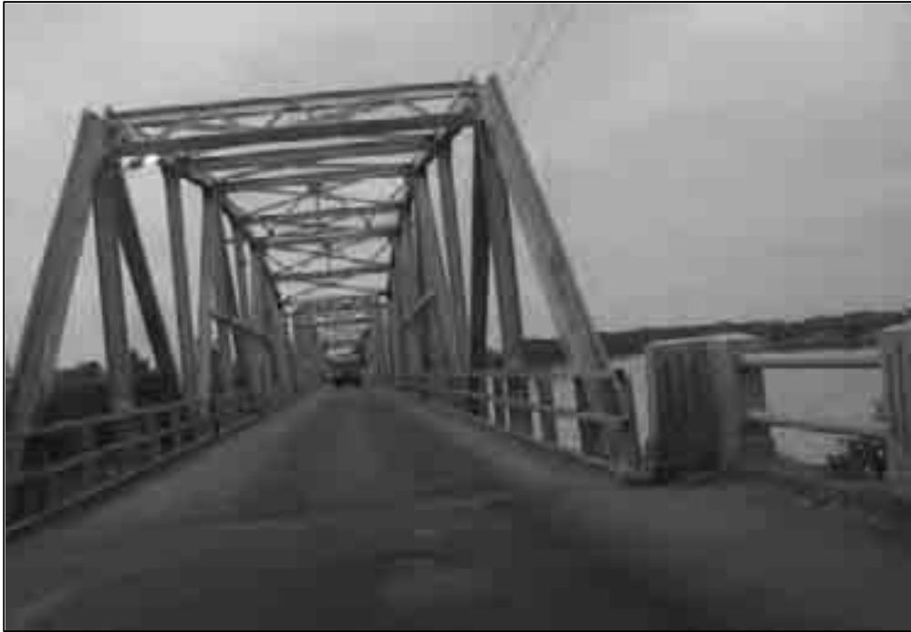
Figure 9-2: Existing bridge over the St George River
