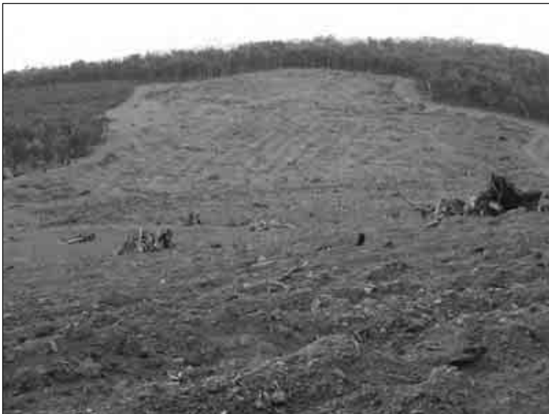
Figure 7-6: Backfilled mined out area with topsoil and reclamation area in background – Saddleback area
