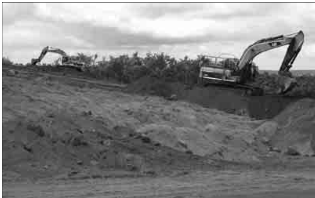
Figure 7-4: Secondary Overburden removal by small backhoe excavators – Saddleback area
