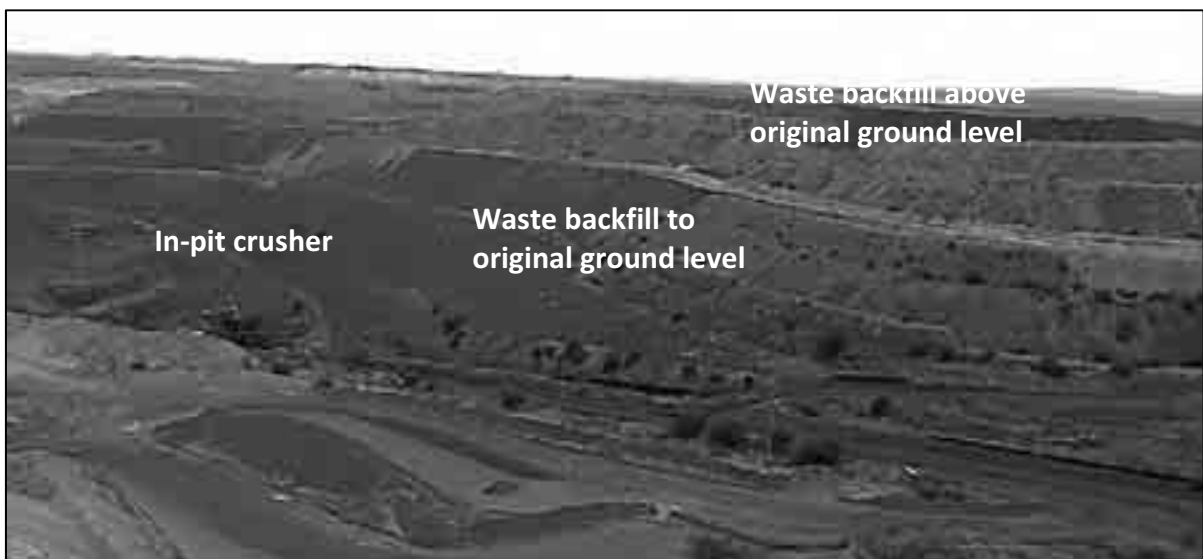
Figure 17 Mamatwan in-pit crusher and backfill Source: CSA Global
