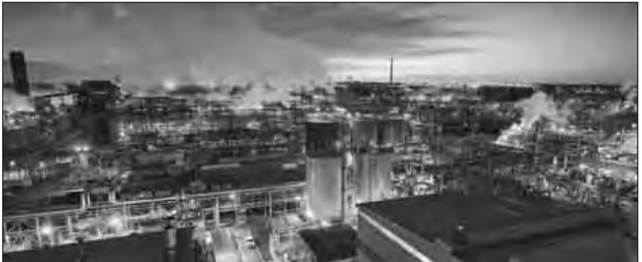
Figure 8-1: Worsley Alumina Refinery
