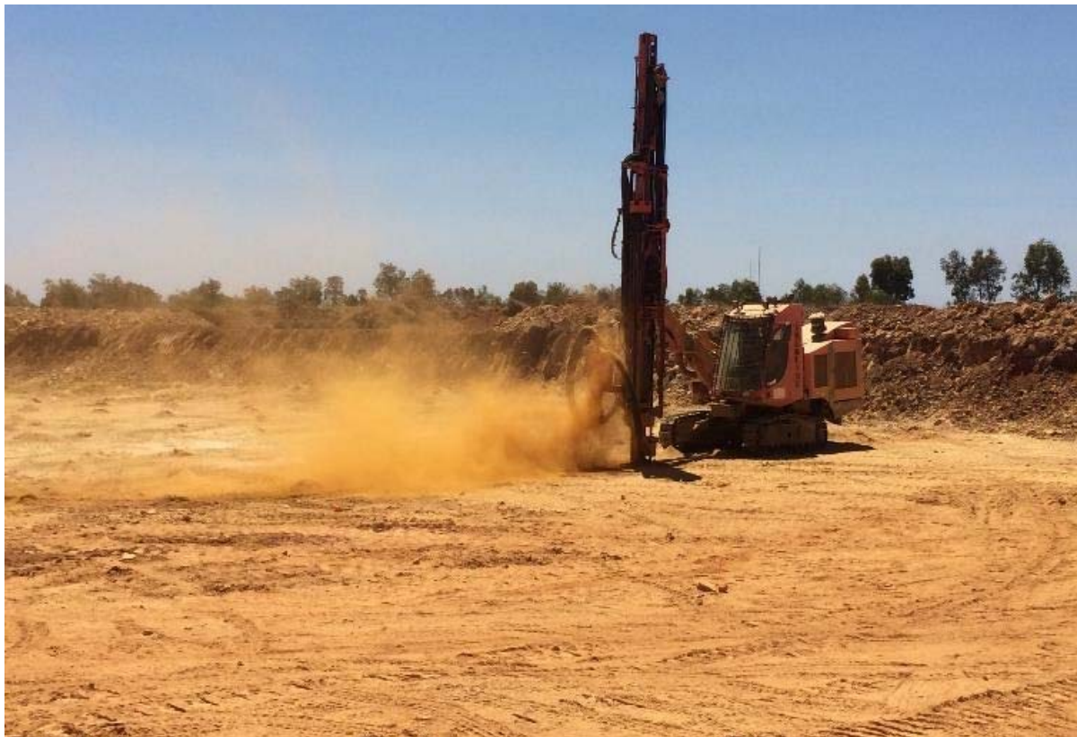
Figure 2. Blast hole drilling at Golden Hind
