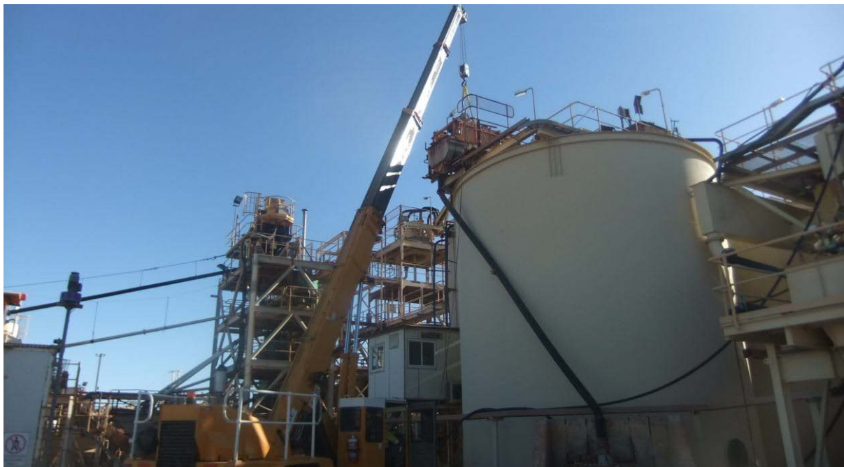
Figure 5. Removing screen above leach-tanks for cleaning and maintenance
