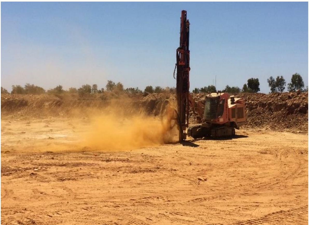
Figure 4. Blast-hole drilling at Golden Hind
