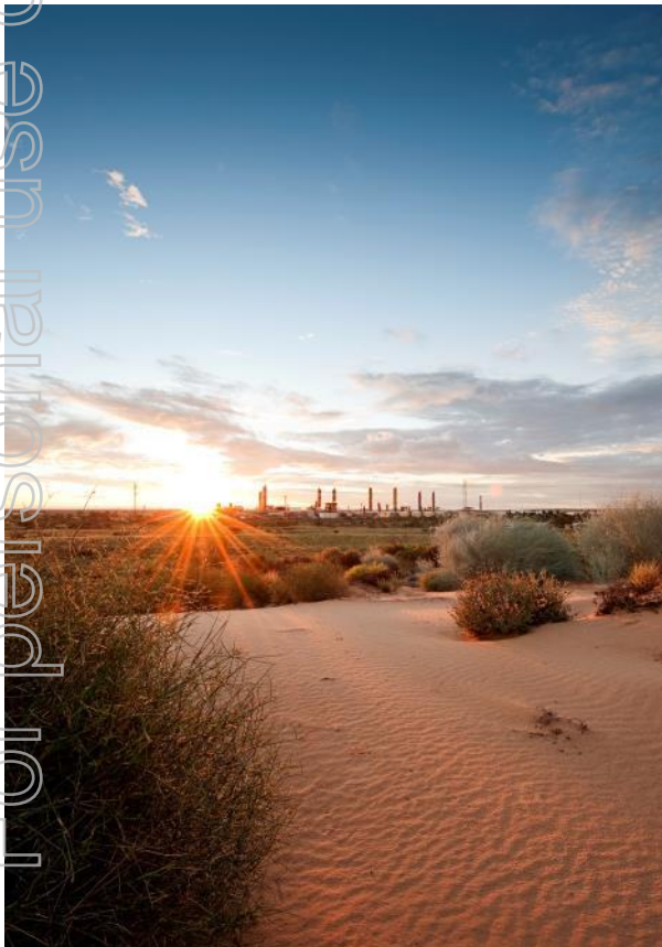
Moomba Plant, Cooper Basin
