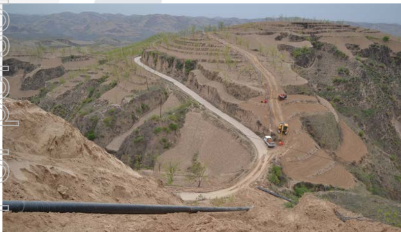
SGE gathering lines being installed
