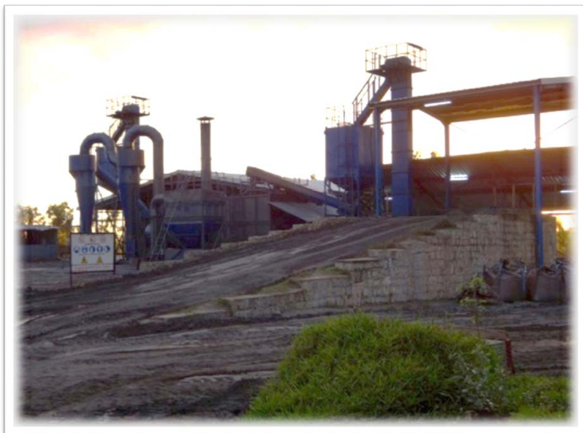
Figure 4: Drying and bagging facilities at Loharano
