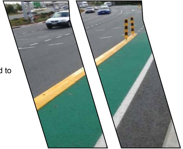
Cinar Kunduz, Project Manager at RoadTek, is very happy with the Saferoads separation kerb solution that directs vehicles to turn correctly and not cut corners and keeps vehicles away from a designated bike lane on a high traffic volume sweeping bend.
