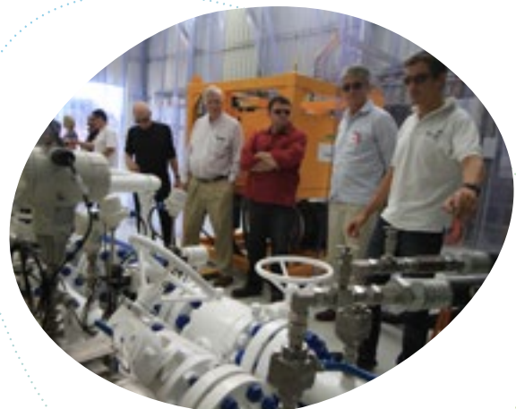
Carnegie's Board of Directors receiving a briefing from Senior Hydraulics Engineer Stephane Dellac at the Perth Project onshore plant
