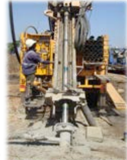
RC / core drilling
