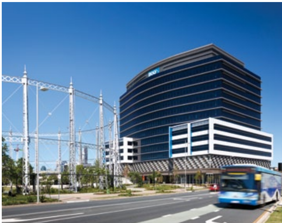
100 Skyring Terrace, Newstead, Qld was officially launched in 2015 with over 50% of the building leased to Bank of Queensland
