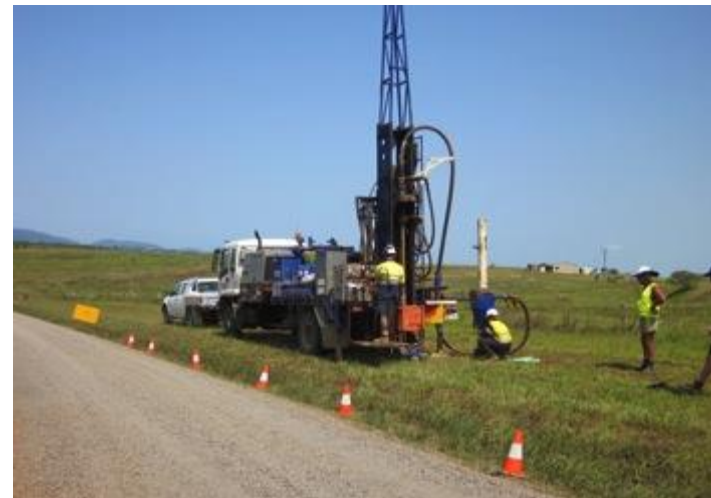
Aircore drilling underway at South Johnstone Project
