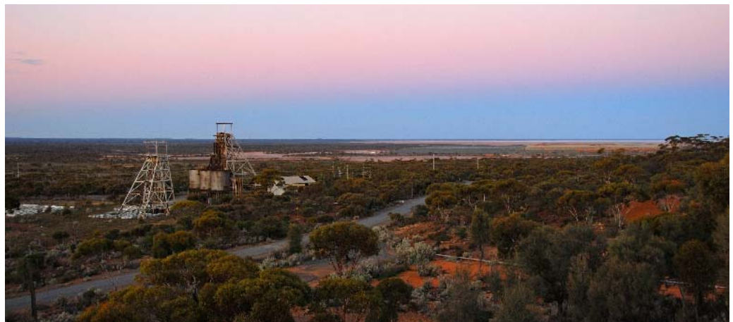
Kambalda Dome – View over Durkin Headframe (photo courtesy of Tanh Doan)
